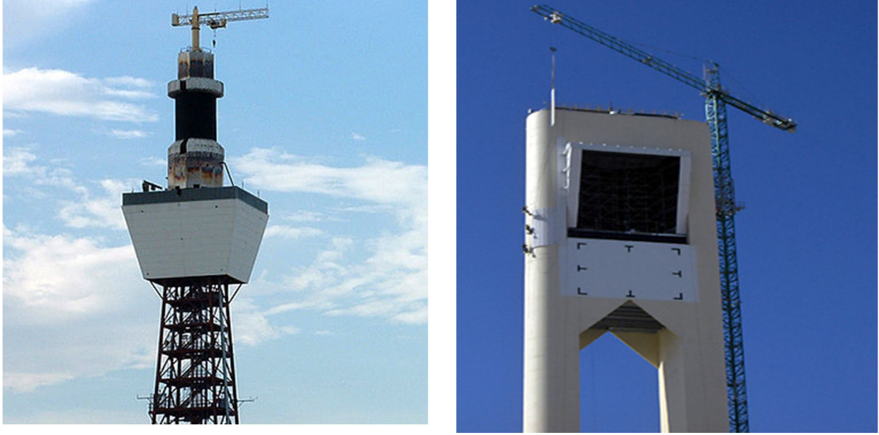
Figure 4-1 Left) External receiver of Solar Two plant. Right) Cavity receiver of PS10 plant
